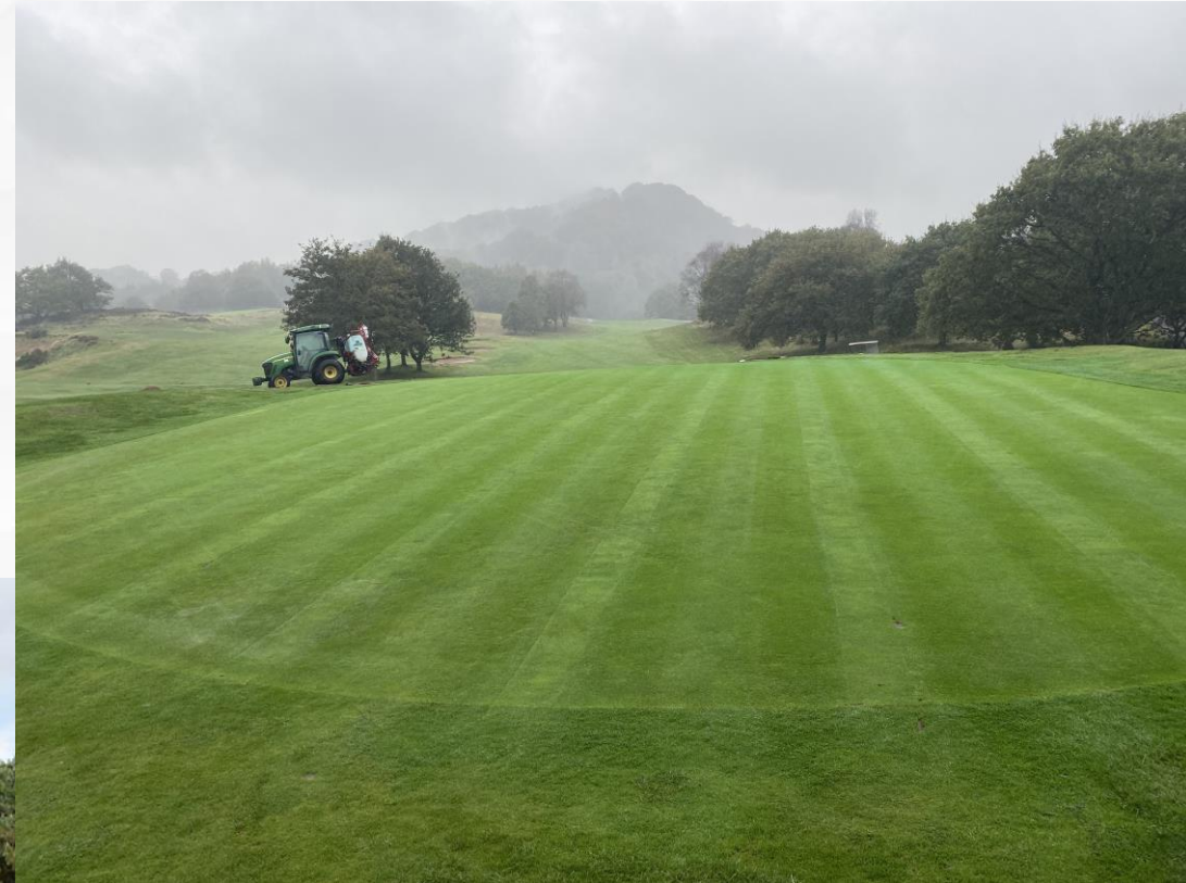
Greens drainage installed
